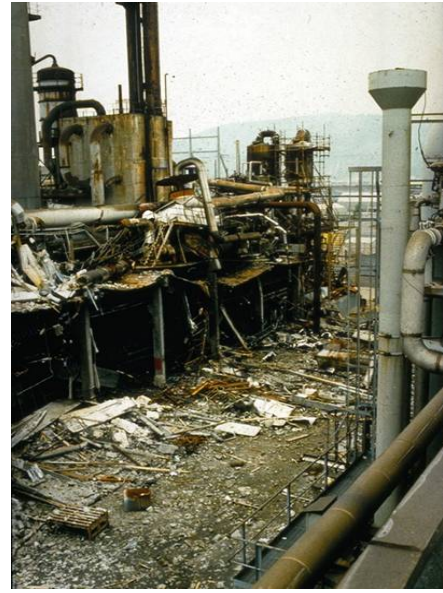
Figure 4 a and b. The wall element of the north wall thrown out
