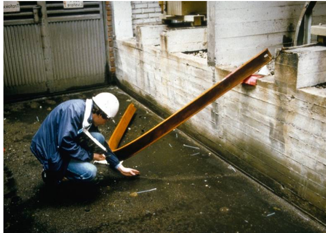
Figure 6. A fragment from the south wall landed 50 m away
