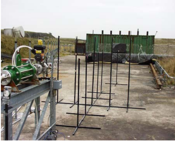
Figure 1(a). Oxygen depletion sensors for low pressure releases (behind release nozzle)
