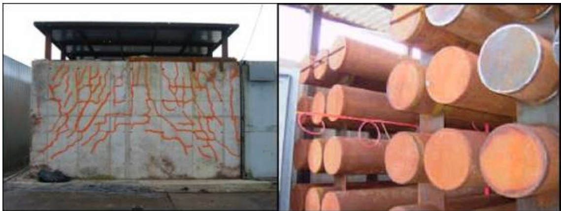
Figure 9: Storage room for high pressure hydrogen (left) and cylinder models (right)
