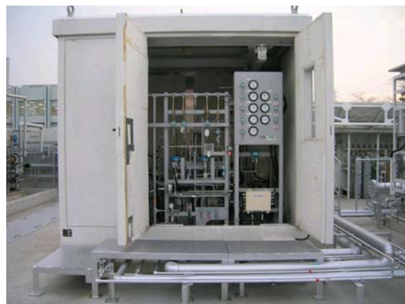
Figure 4. The compressor in the casing
