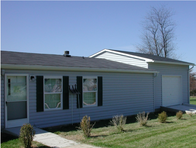
Indoor Environment and Ventilation Test House NIST
