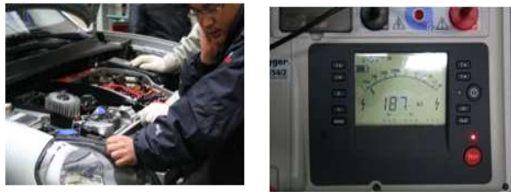
Figure 16. Insulation resistance evaluation.
