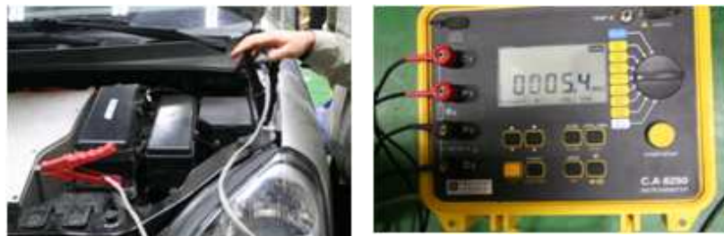
Figure 17. The high voltage box enclosure and the chassis evaluation.
