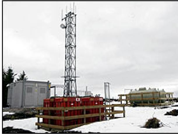
Figure 3. Use of PlugPower GenCore © Fuel System to provide remote power for a telecommunication mast in Scotland (© BBC)
